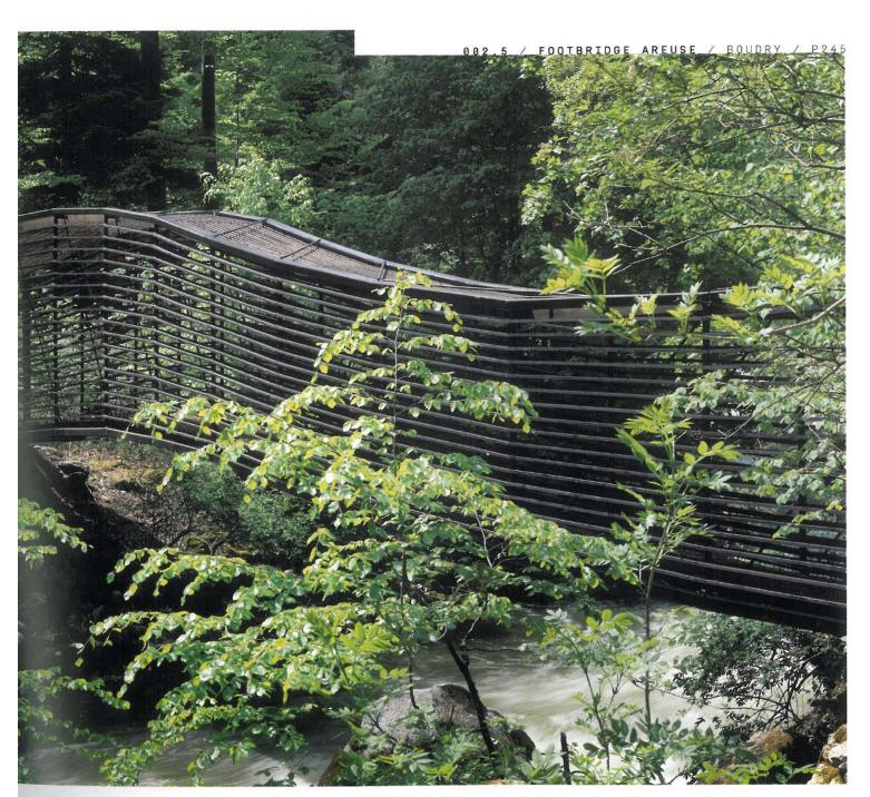
OPPOSITE The shape of the wood and steel footbridge evolved in response to the river bank topography. ABOVE Because of its S-shaped form, the bridge absorbs all structural tension, spanning the river without any supporting elements.
